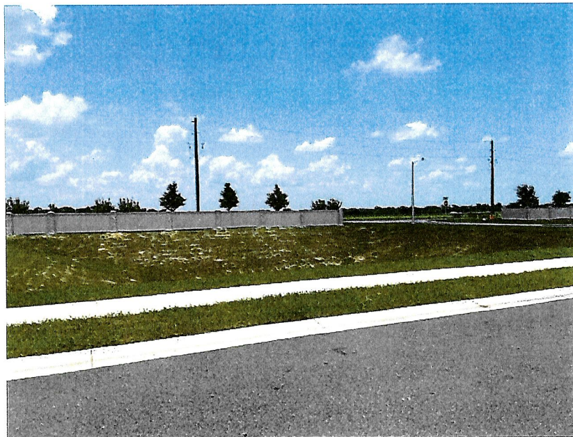
Tract D Cypress Park Estates Phase 2 at Silver Palm Drive and Buttonwood Way
