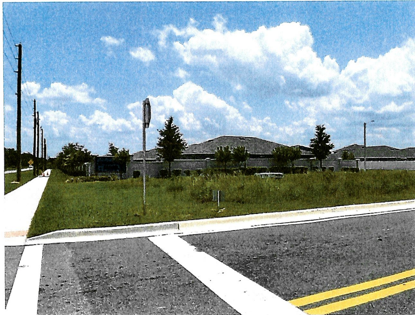
View of Tract A Cypress Park Estates Phase 1 common area at Baker Dairy Road and Bice Grove Road
